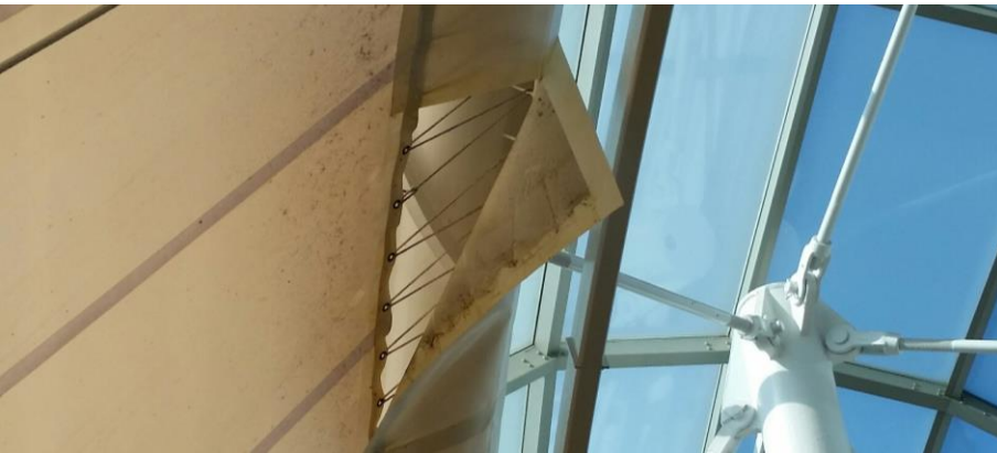
Detail showing some of the wear/ damage to tent fabric
